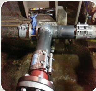
▲ Netherland desalination treatment facilities
