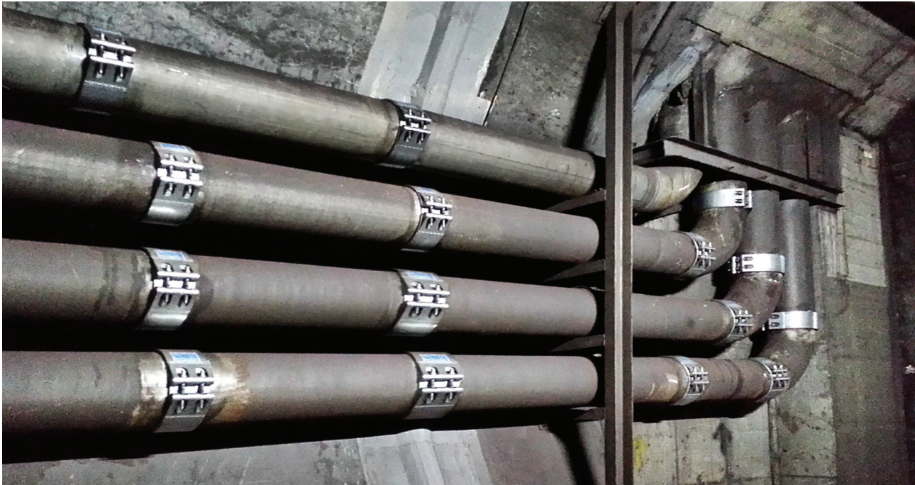
▲ Underground drainage repair(Maintenance) works
