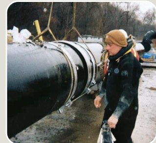
▲ UK: district heating work
