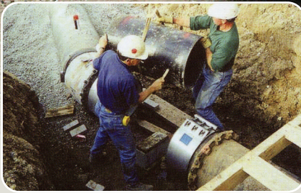
▲ Repair work for pipes replaced underground
