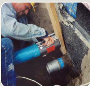
▲ U.S.: sewerage repair work
